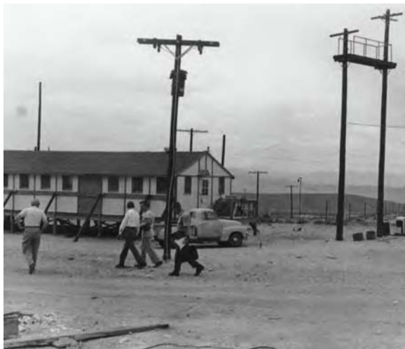
Control Point (CP) building, moved from Los Alamos.
